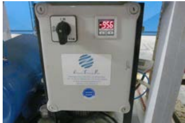
Figure 3.2.15. setting for vacuum pump.
